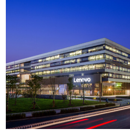
Lenovo Headquarters Beijing, China
